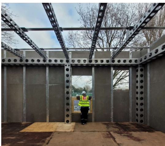
Above: A worker stands in a structural aperture.
