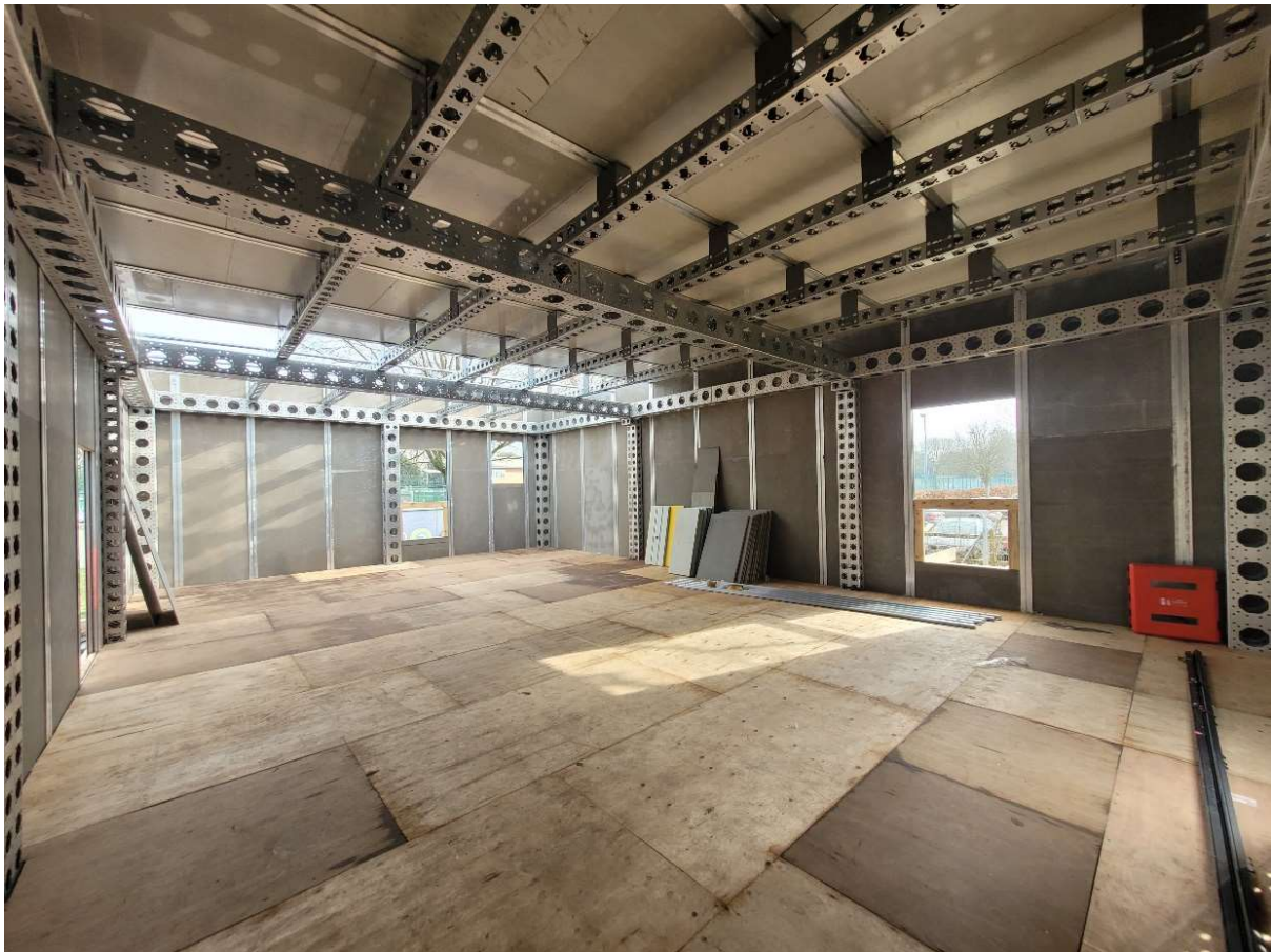
Above: Working towards completion, the image shows structural openings, a 75% finished roof, completed walls and floor, and a stack of materials ready to be fitted to the roof.
