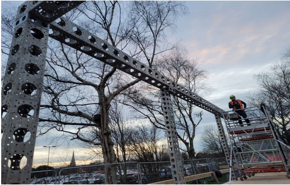
Above: worker standing triumphantly in a mobile scaffold tower next to a series of columns and transoms which they have just assisted in building.
