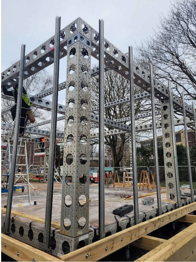
Above: Completed structural Frame and more extrusion.
