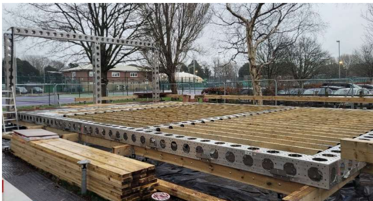
Above: Progress shot, showing progress at the end of build day 1. Showing a full ModTruss floor raft, Joists, insulation started in far extremes, thermal barrier, and ply flooring, and the first vertical elements shown.
