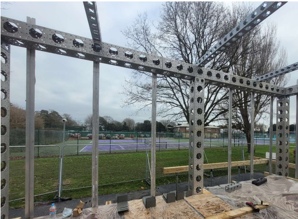
Above: Extrusions which hold the wall and ceiling cladding fitted to a finished structural frame.
