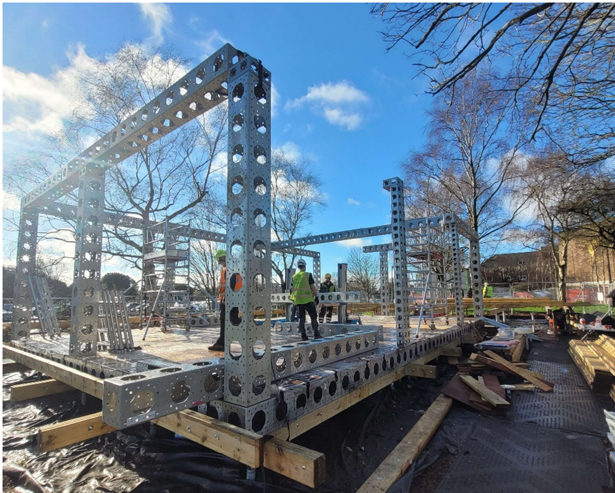
Above: The structure starting to take shape with most of the exterior columns, transoms and ledgers in situ.
