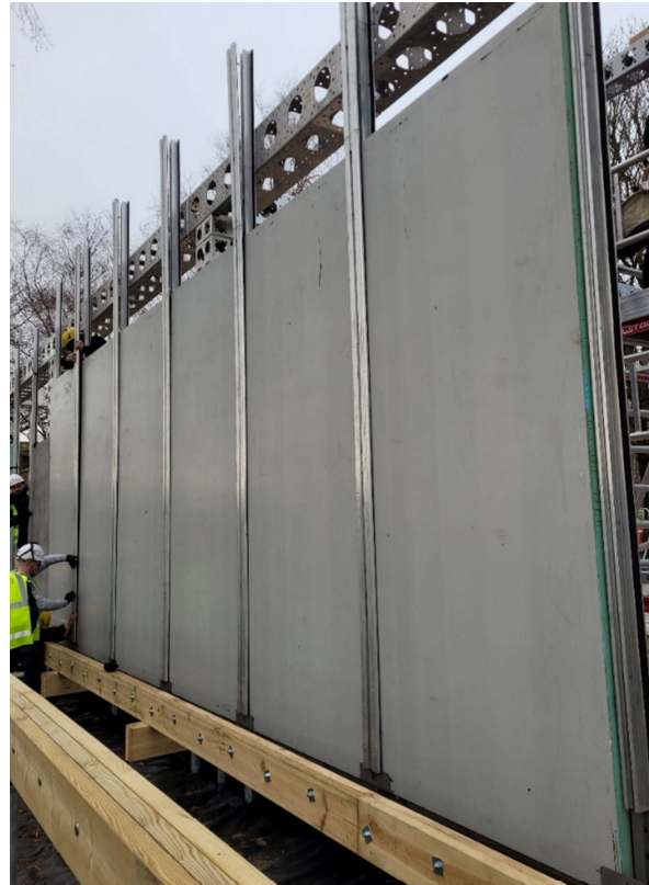
Above: Panels being fitted between the innovative Triple E Curtain wall extrusion.
