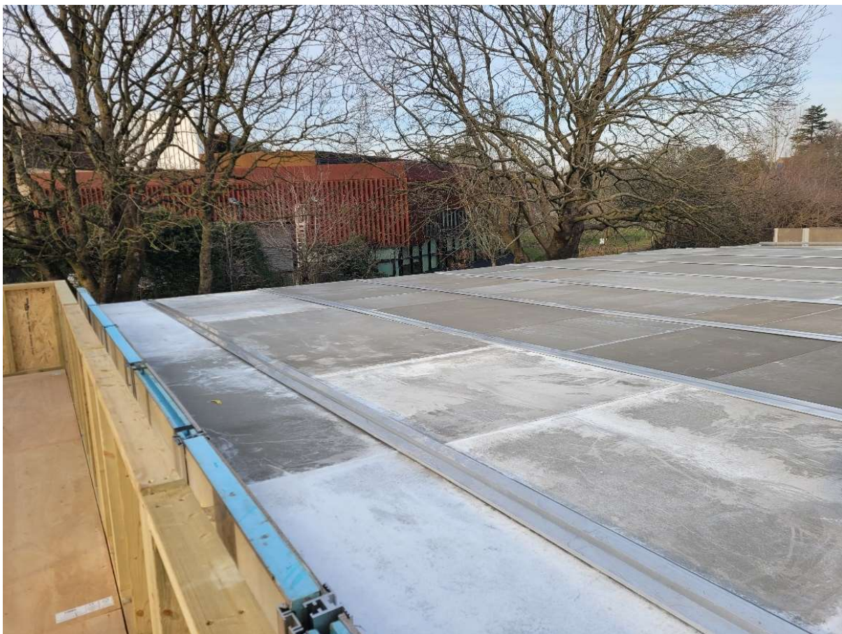
Above: Finished Roof cladding, awaiting the roofing contractor to install weather tight seal and drainage system.
