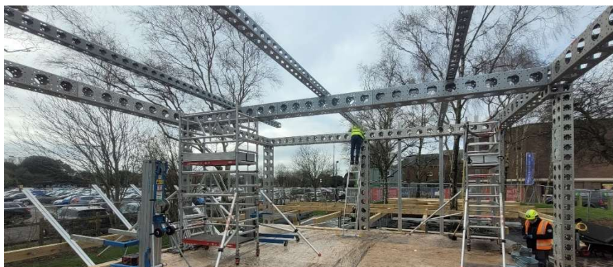
Above: Workers assembling the Columns, Transoms and Ledgers, using Scaffold towers, ladders and Genie material lifts.
