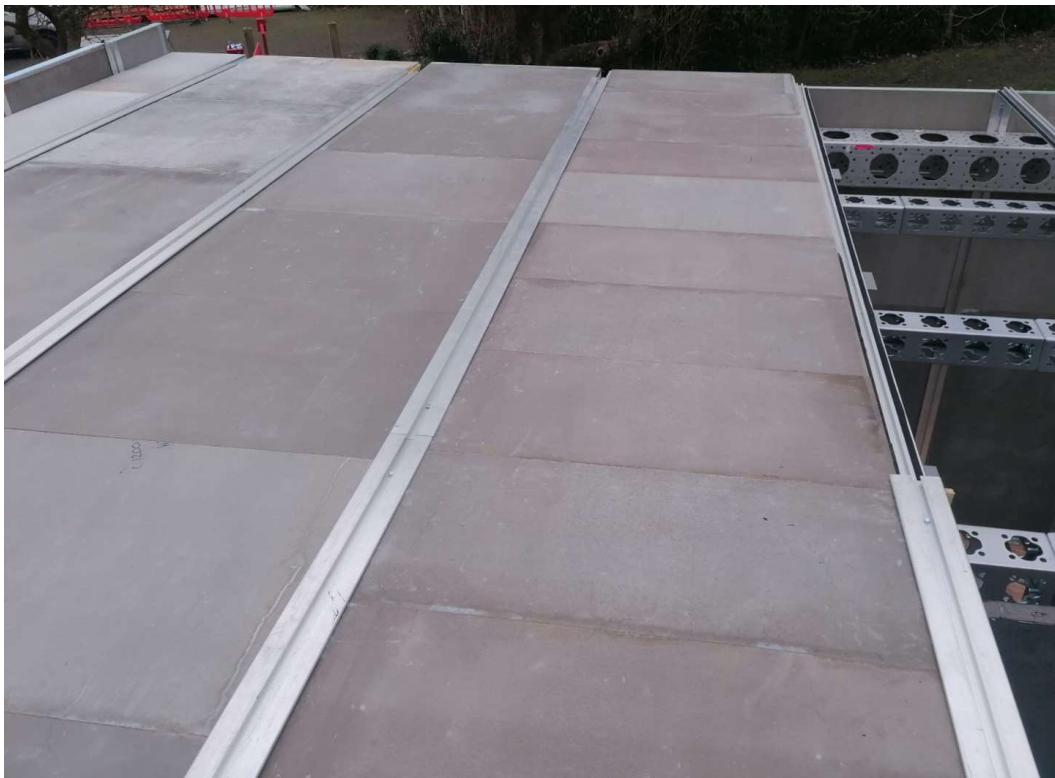
Above: Roof panels being fitted between the innovative Triple E Curtain wall extrusion.
