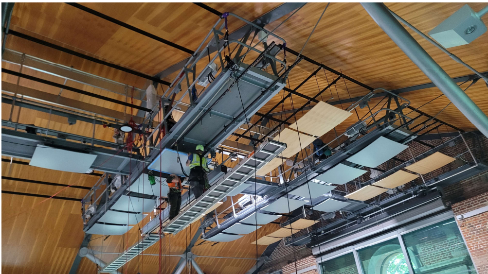
Works Underway Transforming the Lighting Bridges with Acoustic Reflectors
