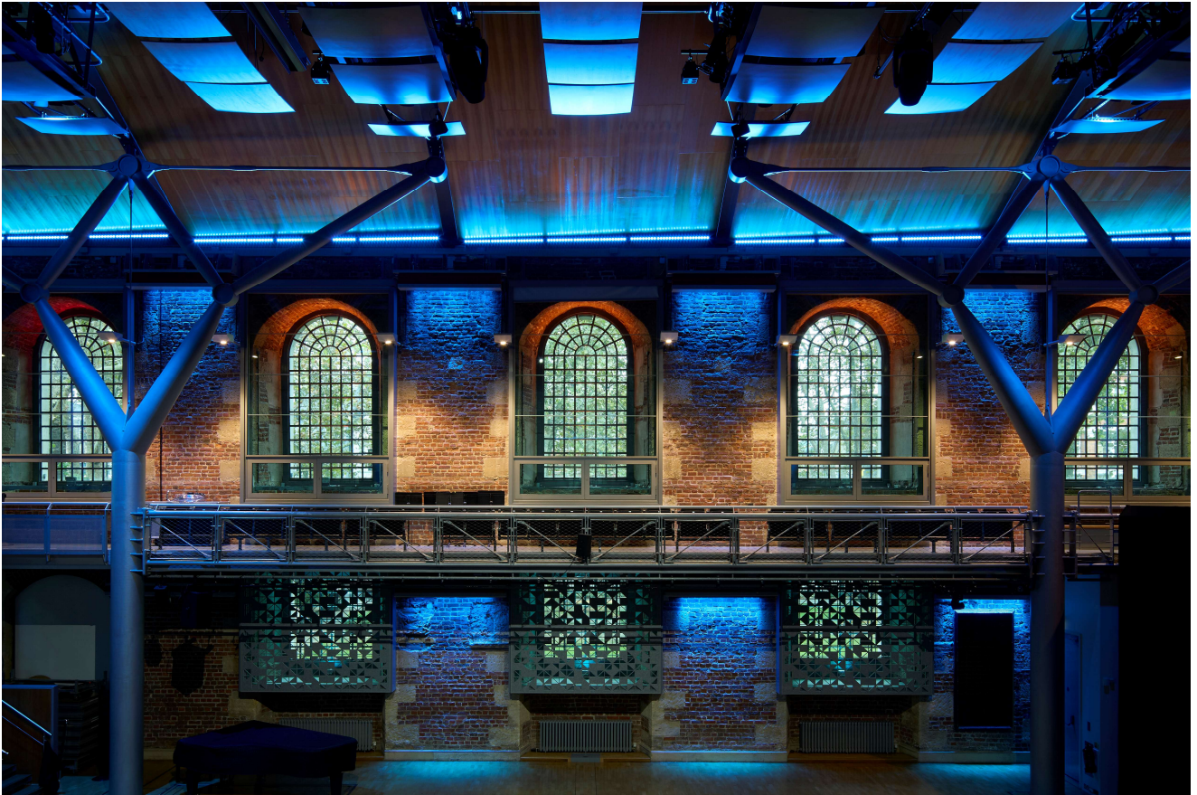
Interior View of South Wall – Jerwood Hall, Showing Acoustic reflectors in the roof, Retracted Acoustic banners to the wall and a moody blue lighting with large windows as a focus to the image. © David Levene
